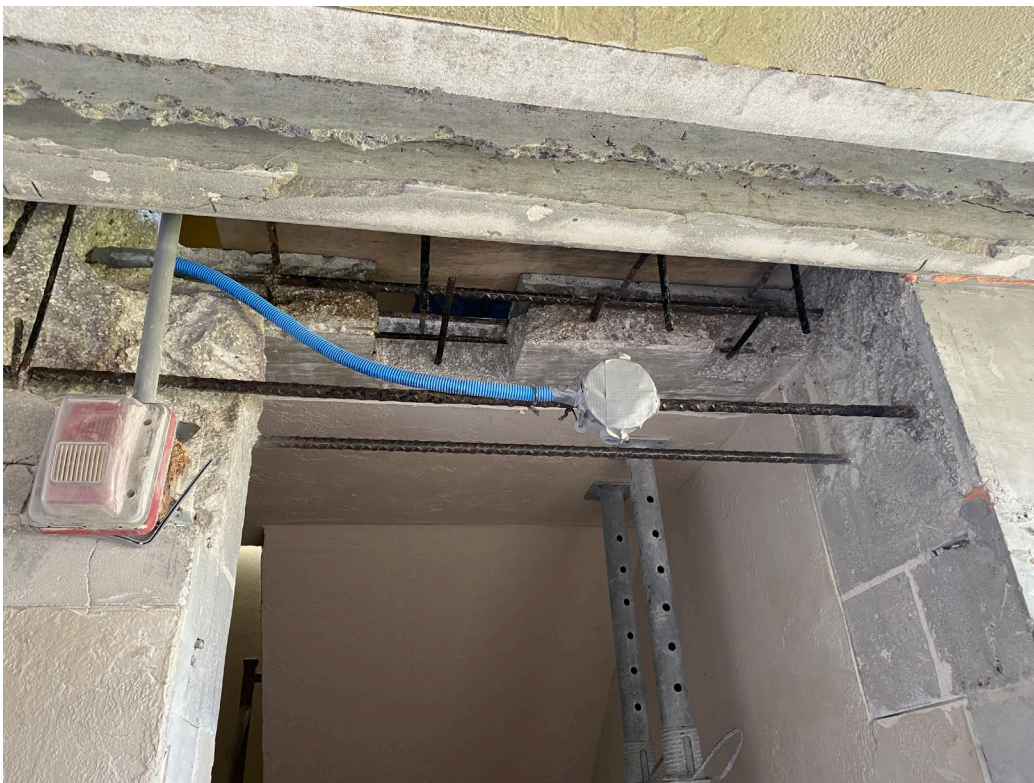
Picture 2: 1 st floor stairwell header repair
