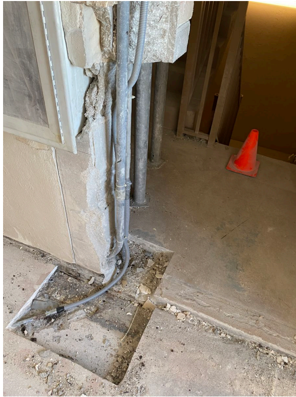
Picture 1: 1 st floor jamb repair
